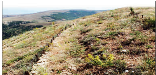
Picture 3: Dump area rehabilitated with hydroseeding application and afforestation program
