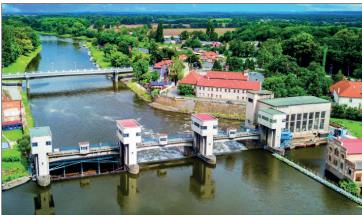
Picture 18: Hydropower plant in Brandýs nad Labem
