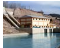
Resadiye Cascade 64.3 MW; 3 HPPs
