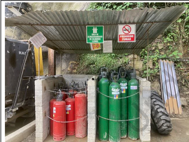
Photo 52: Gas bottle storage at tunnel portal
