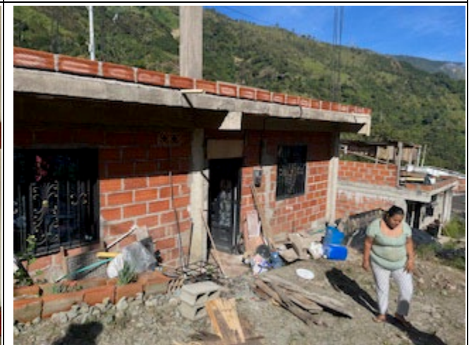
Photo 6: Newly built home for resettled family in San Andrés
