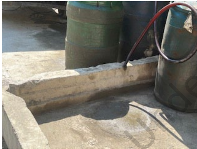
Photo 46: Improved oil containment, follow-up visit January 2024
