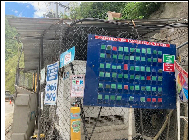
Photo 54: Control of workers' presence in tunnel
