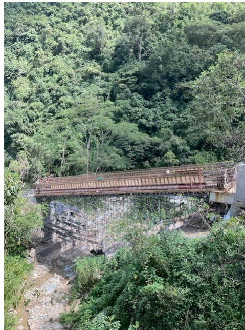
Photo 44: Bridge on access road from highway to powerhouse
