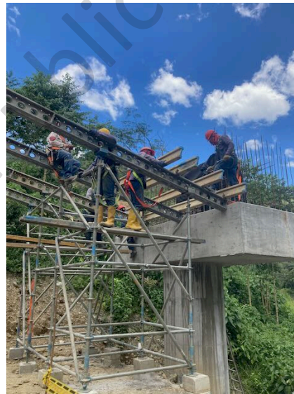
Photo 65: Workers with PPE for work at heights
