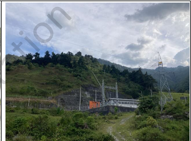
Photo 3: Powerhouse of Celsia's upstream San Andrés HPP
