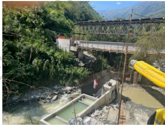
Photo 47: Improved retention of sediments at upper tunnel portal, follow-up visit January 2024
