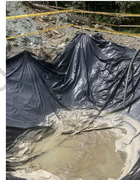
Photo 57: Temporary sediment trap at lower tunnel portal
