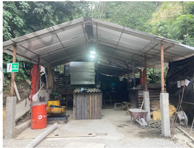
Photo 41: Equipment storage and worker rest area at lower tunnel portal
