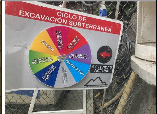
Photo 36: Signage for current stage of tunnelling activities
