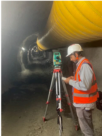
Photo 55: Control of alignment in tunnel construction
