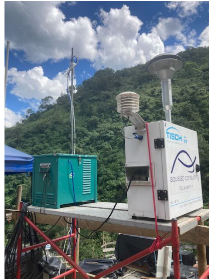
Photo 62: Monitoring equipment at powerhouse construction site
