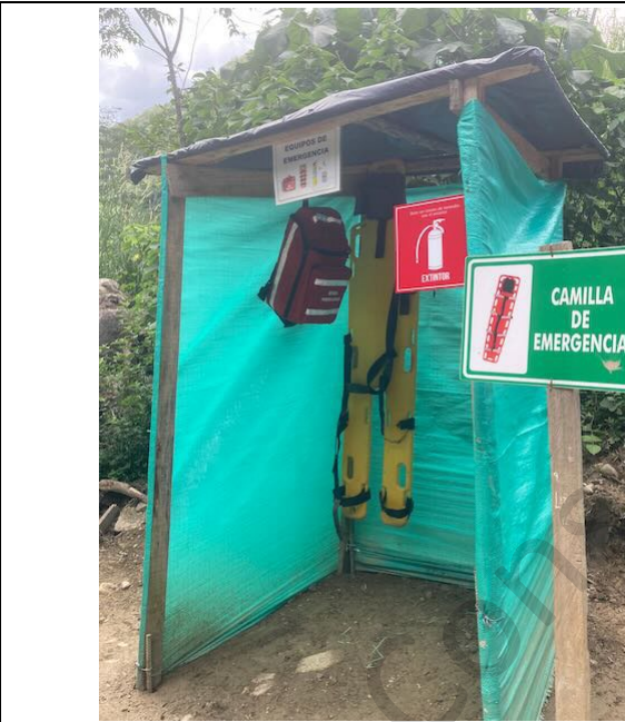
Photo 50: Emergency equipment at powerhouse construction site
