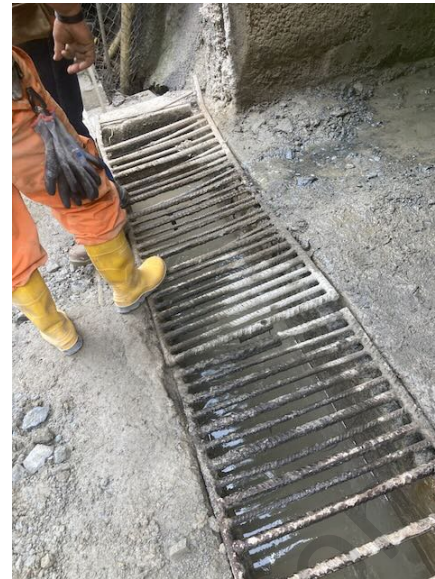
Photo 56: Drainage at lower tunnel portal
