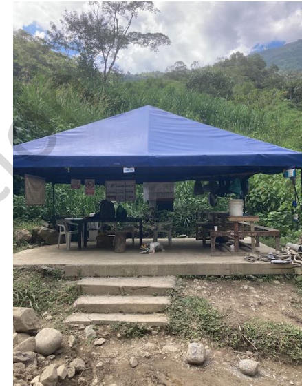
Photo 63: Rest area for workers at powerhouse construction site
